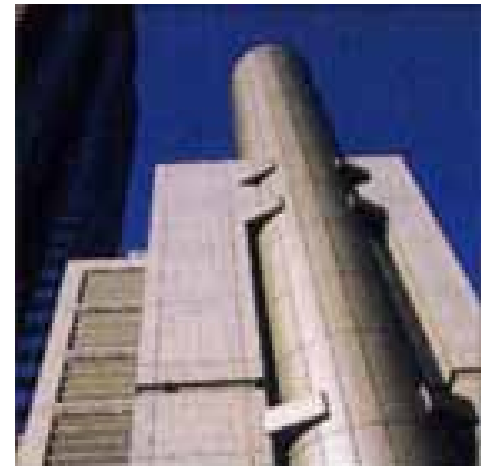
Nishi-Shinjuku Tokyo Gas Building
